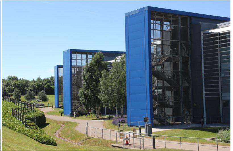
Locker Gladstone PC architectural mesh installed at The Met Office in Exeter.
