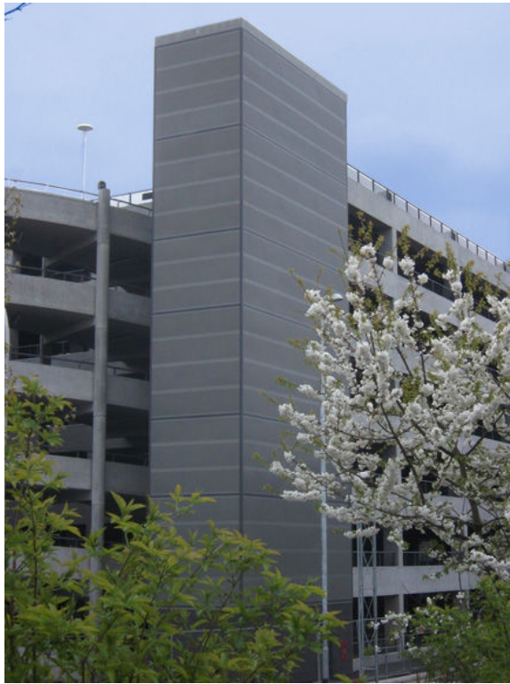
Shaldon 4/8 perforated metal installed as stair tower cladding at Gatwick Airport.
