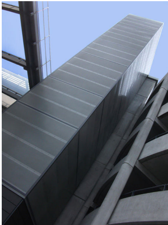
Shaldon 4/8 perforated metal installed as stair tower cladding at Gatwick Airport.
