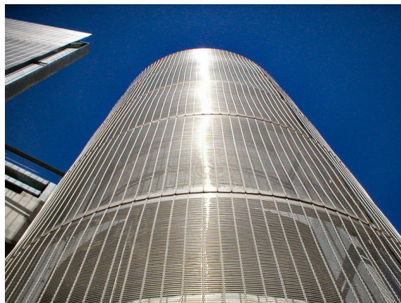
Gladstone PC 80/10 architectural mesh installed as car park cladding at Cork County Hall Car Park, Cork, Eire.
